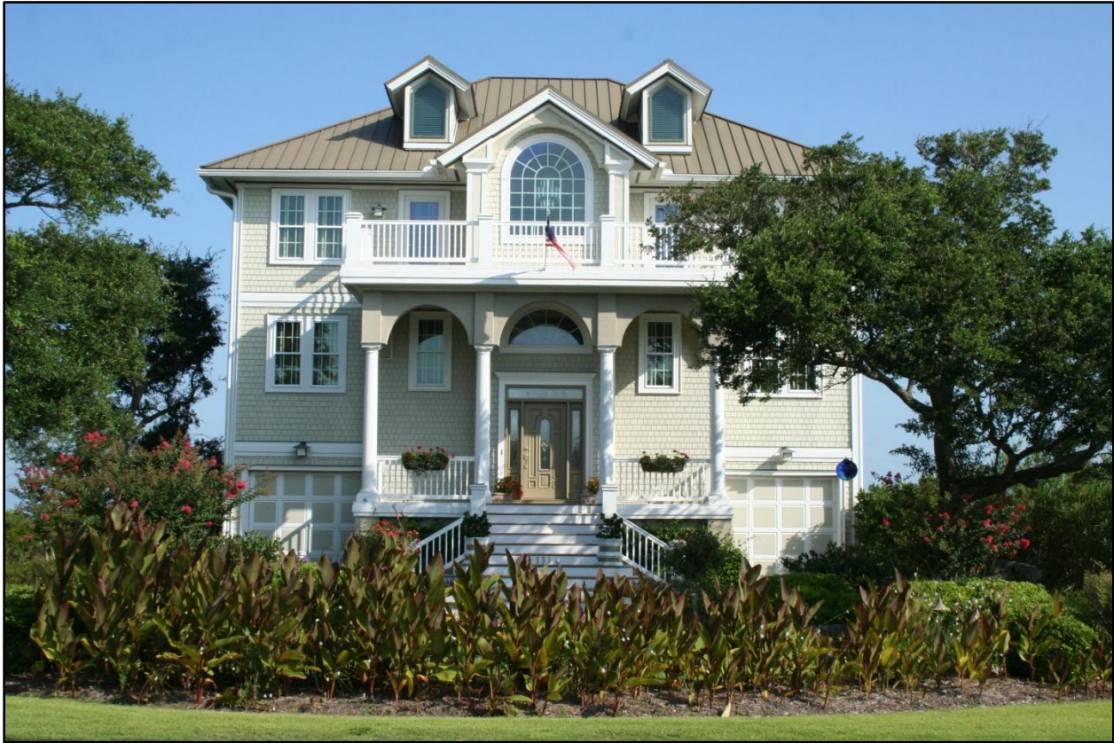
Street view of home with breakaway walls and elevated first floor
